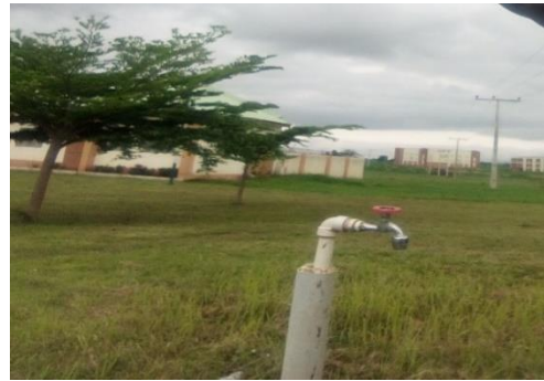
Tape Water within the project
